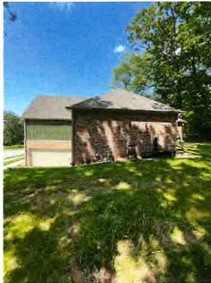
Southwest side of home
