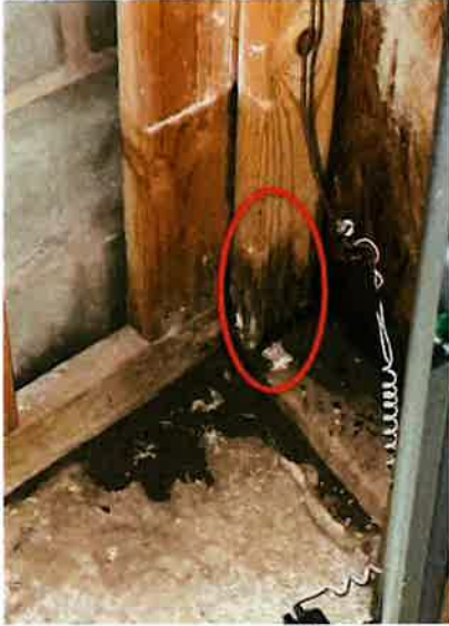
Garage SW wall
