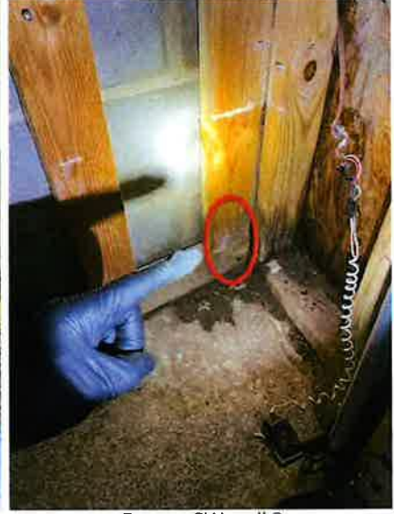
Garage SW wall 2
