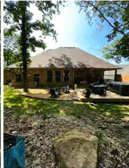
Southeast side of home
