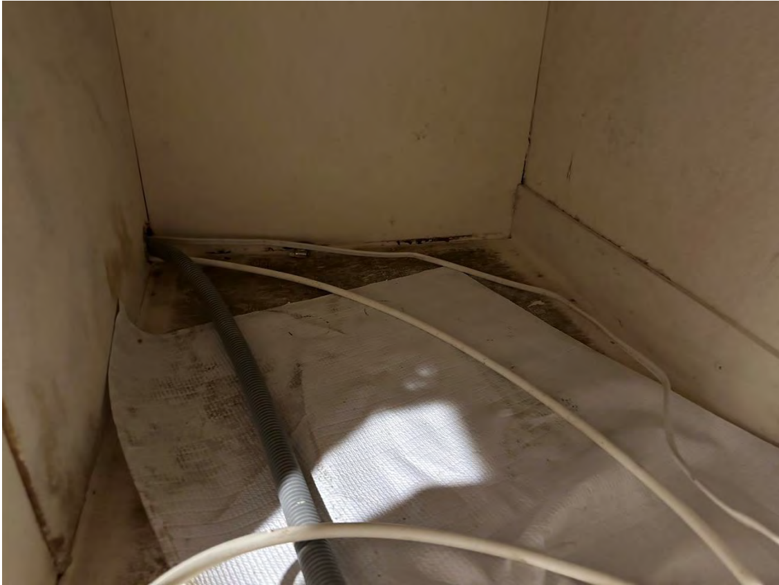
Photo 4. View 2 underneath kitchen cabinetry housing the kitchen sink illustrating visible mold growth
