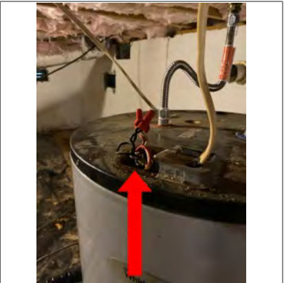
Exposed electrical wiring
