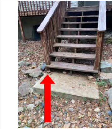
Wood deterioration
