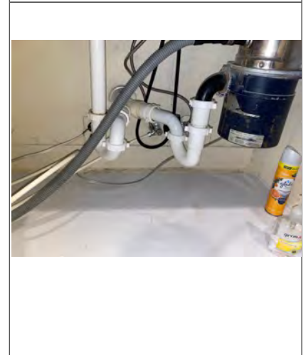
Missing vent cover mentioned for your reference
